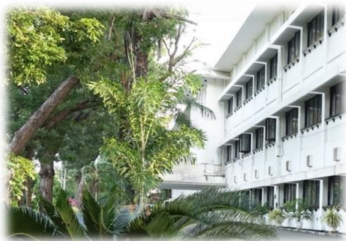
Figure 4: West wing of the Faculty
