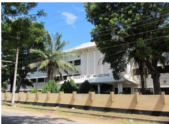
Figure 2 : Entrance to the Faculty building
